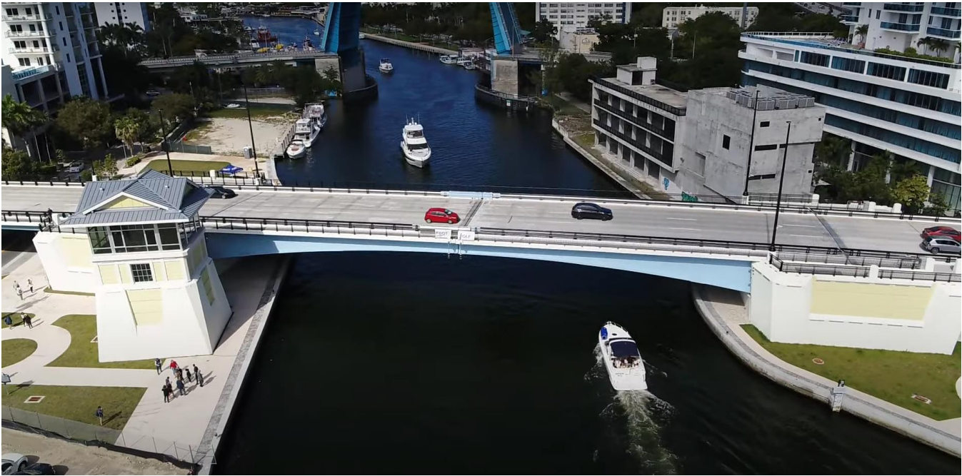
First Street Bridge
