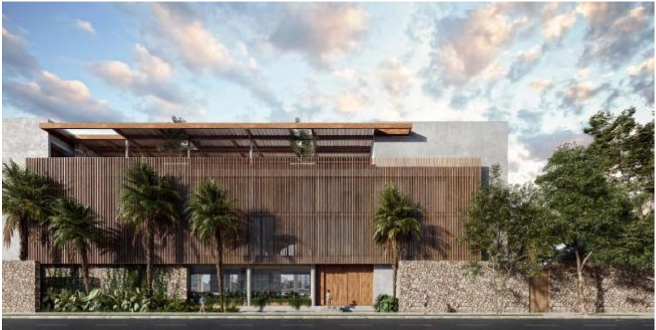
View from River Drive
